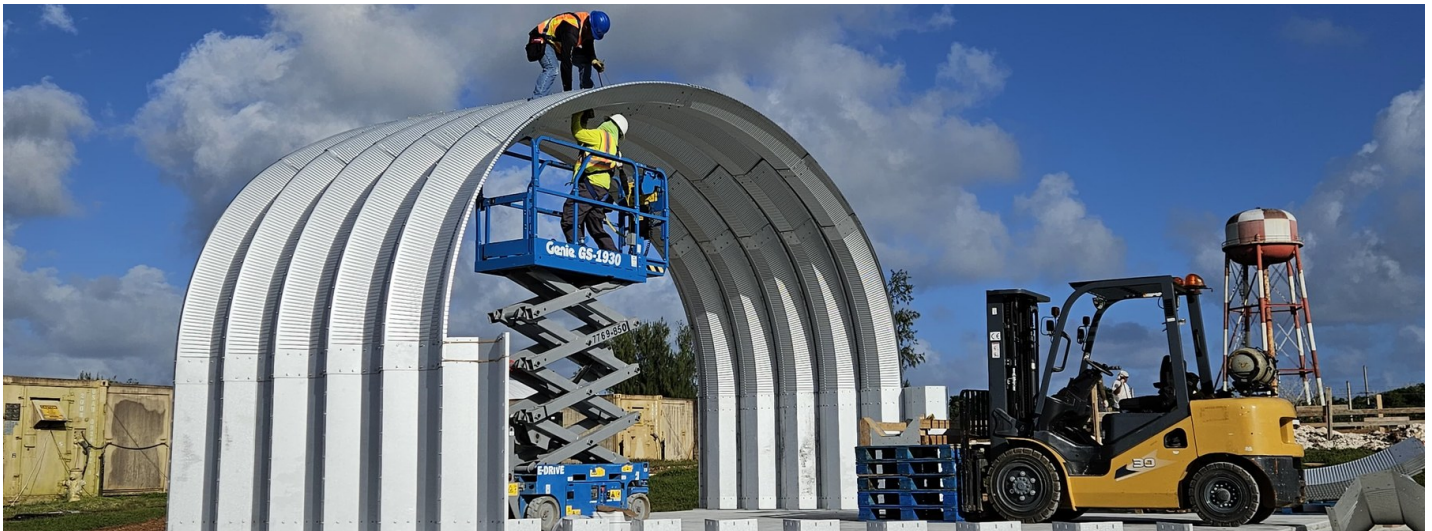
Arch panels going up on site — bolted, panel by panel, off the base connectors.
